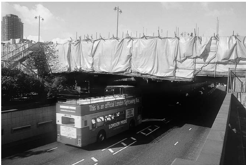
Figure 11.6 Containment of blasting and painting operations in a sensitive area.
