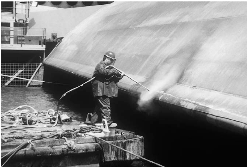
Figure 3.8 Ultra-high pressure water blasting on London's Thames Barrier.
