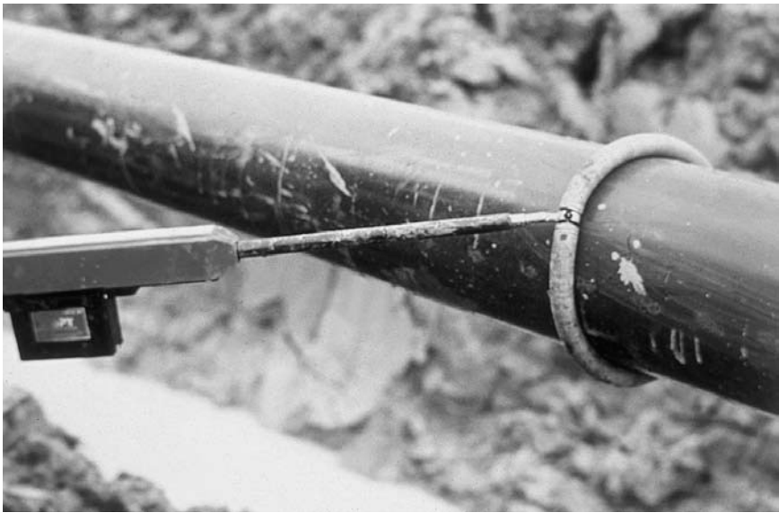
Figure 6.2 Pinhole testing of coated pipeline.
