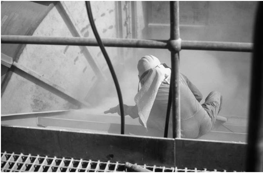
Figure 3.5 Air blast-cleaning on site.
