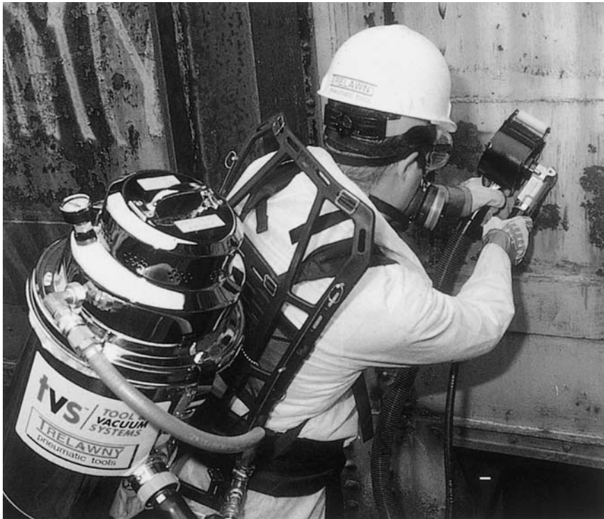
Figure 3.4 Vacuum shrouded coatings removal, mechanical cleaning system.
