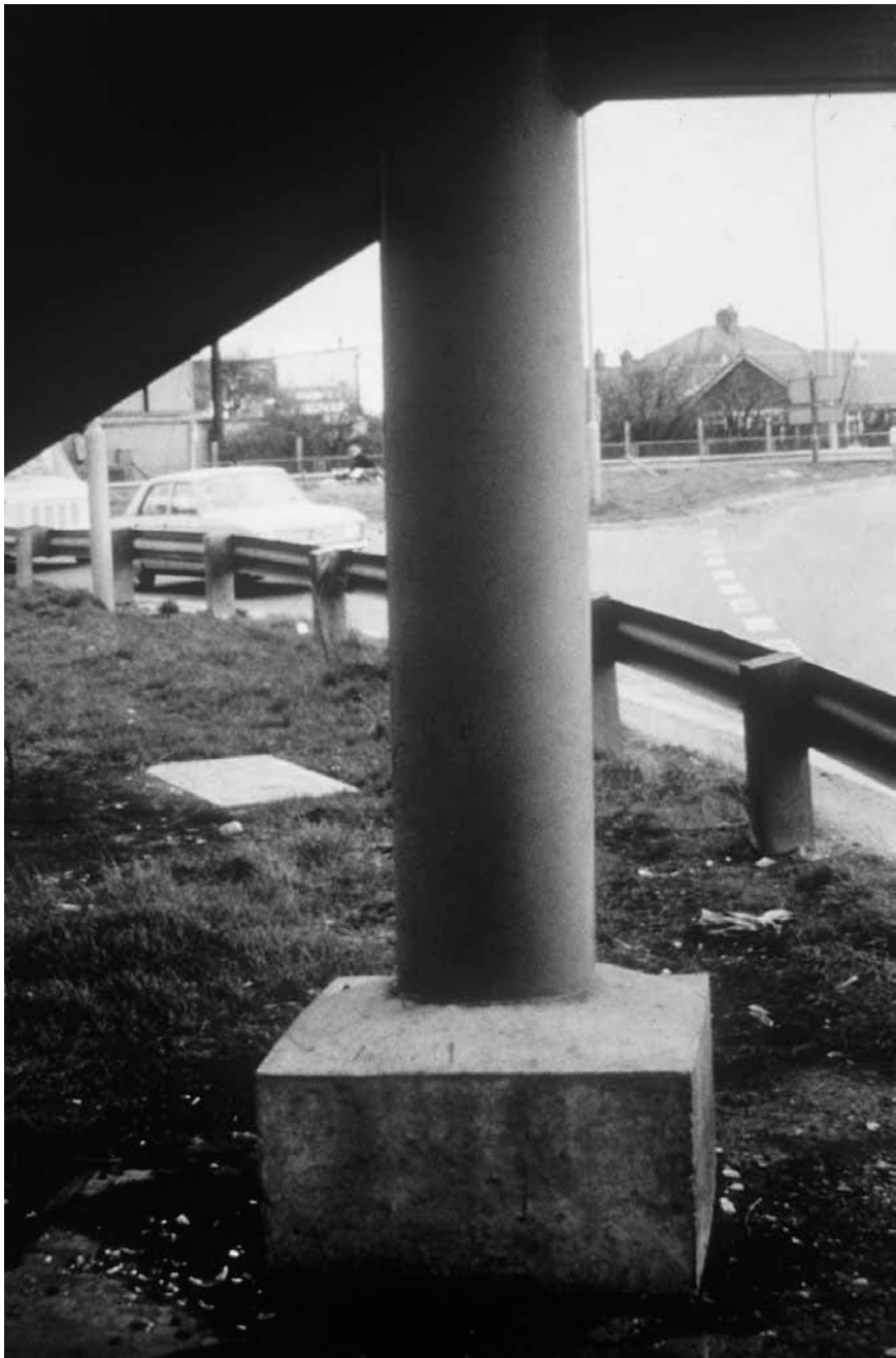
Figure 10.6 Concrete plinth to protect steel at ground level.
